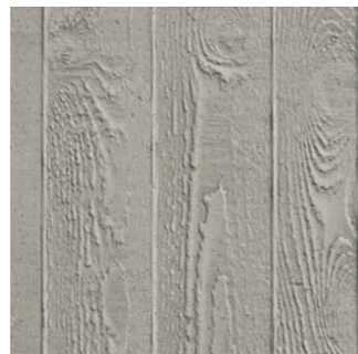
Brettschalung | timber formwork
